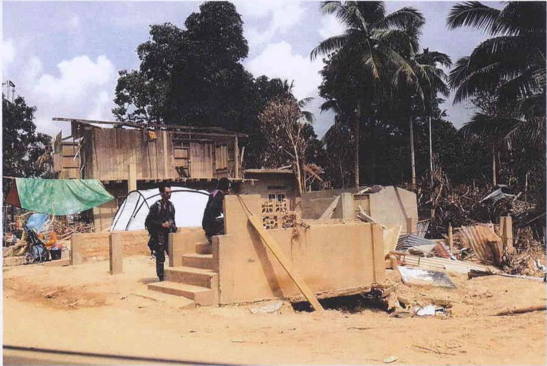
Remains of the flood – some pillars and staircase of homes
